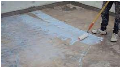
Fig.1. Application of Latex Bonding Agent
