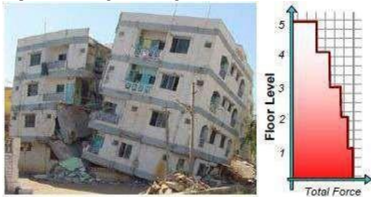
Fig-Total horizontal earthquake force in a building increase downwards along its height
