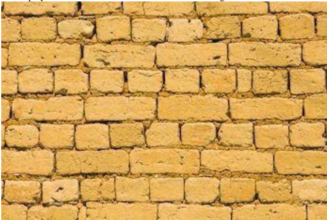
Fig. 1: Brick work in mud
