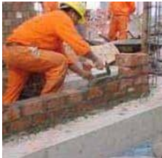
Fig. 6: laying bricks
