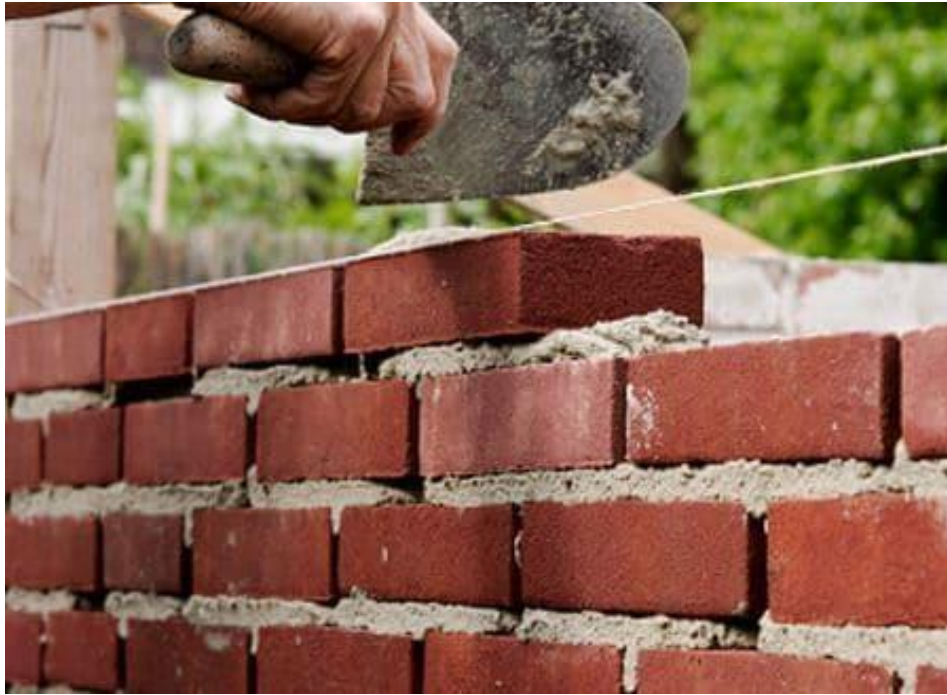
Fig. 2: Brick work in cement
