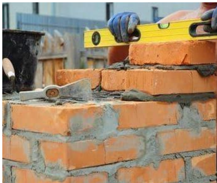
Fig. 8: Checking level of brick masonry
