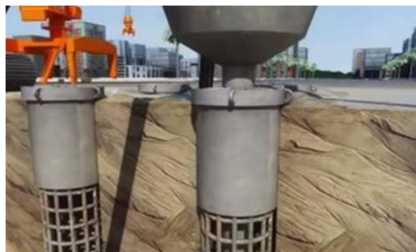
Fig.4. Diaphragm Joints by Disposable PVC Pipes
