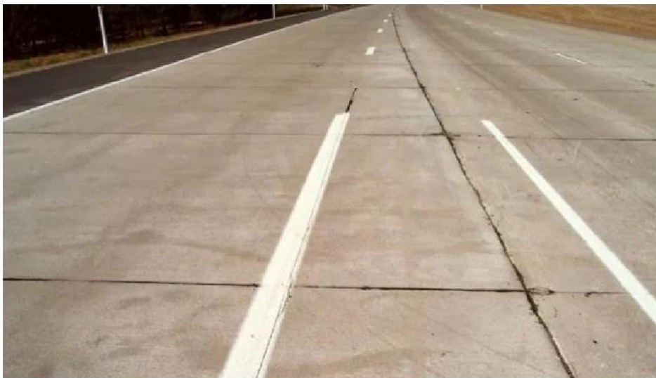
Contraction Joint in Concrete
