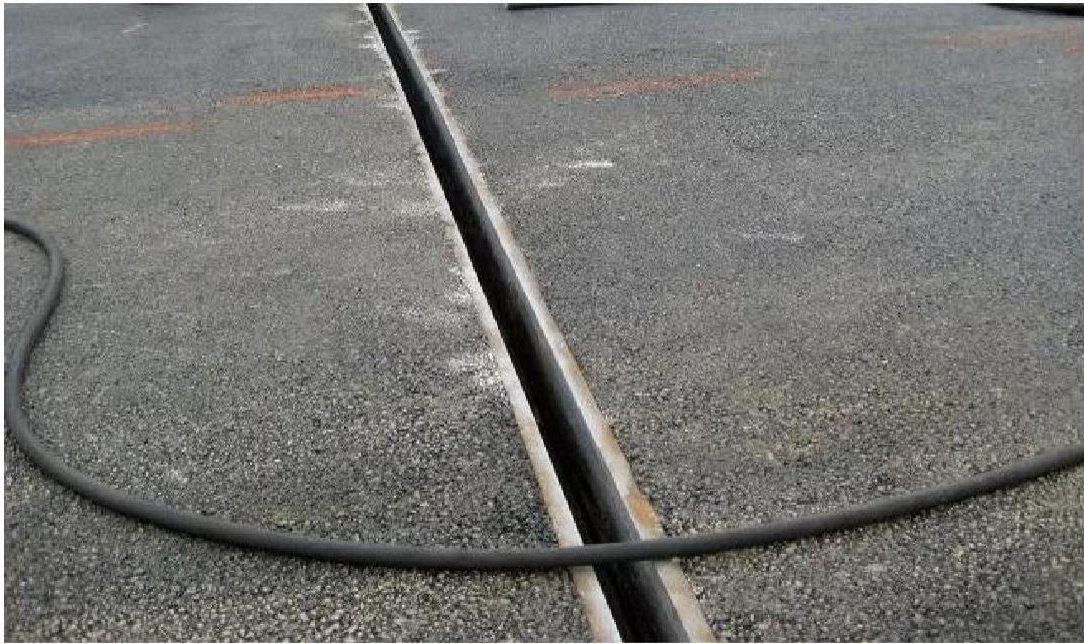
Expansion Joint in Pavement
